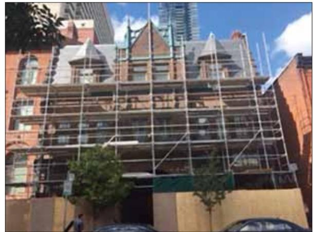
The scaffolding is up, and the front façade conservation project will begin shortly! The work includes repairing and cleaning the stone and brick, repairing downspouts, painting eaves and window sills and more.
